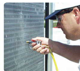
Blow off coils with the Sludge Sucker® Blowgun
