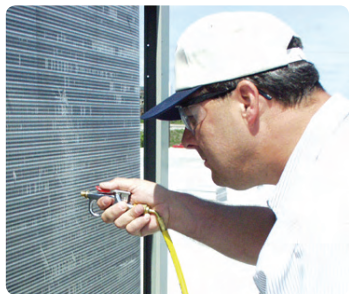
Blow off coils with the Sludge Sucker® Blowgun
