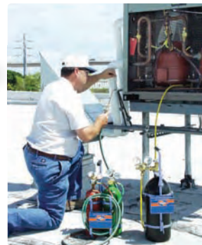
Purge & Pressure Test an A/C&R System
