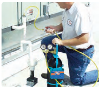
Clean condensate drain lines with the Sludge Blaster®
